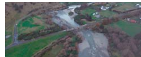
Twin Bridges: Follow the rail from the north.
