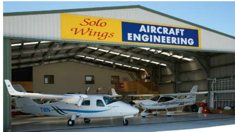
Solo Wings new hangar complex at Tauranga. The company is a recognised official Tecnam Service Centre and will be caring for Bay Flight Aviation's new P2006T Twin.
