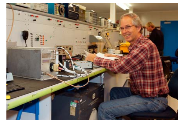
Hawker Pacific's new AeroFlex Test Bench installed at Ardmore.
